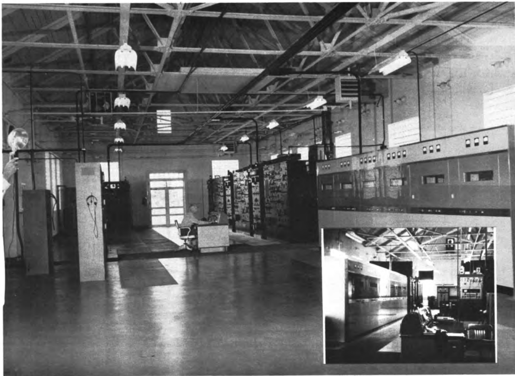
The Transmitter Building at South Chatham is located on a 72 acre plot, mostly marshland bordering Nantucket Sound off Forest Beach Road. At this location are rhombics, "fishbone" and sloping antennas, including traditional lattice type steel tower 400 feet high. This large picture was taken in 1948 and is taken from the rear looking toward the front door. Picture from the RCA collection and furnished by Ed Hammons. The smaller insert at bottom right was taken July 1 1980 and shows considerable more equipment over the years. It was taken from the opposite end of the building. Picture is from the collection of Bill Ryder. In the larger picture, Frank Kremp is shown at desk control unit in center.
